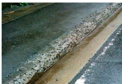
Fig.2 Salt Scaling of Concrete due to the Influence of the Deicing chemicals
