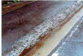
Fig.2 Salt Scaling of Concrete due to the Influence of the Deicing chemicals
